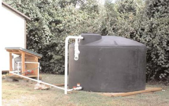
*The District collects water off a 640-sq. ft section of roof. The water is gravity-fed into a 1550-gallon black polyethylene tank, which becomes nearly full after a 4 in. rain. We chose this lightweight, dark-colored tank in order to prevent the growth of algae. It measures approximately 7'-6" in diameter by just under 6'-0" high.*
