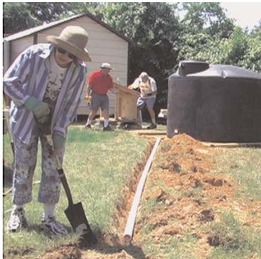
Mary Helen Quinn, Master Naturalist, helps dig the ditch for the PVC piping. Due to drainage issues, the tank needed to be located away from the building and downspout.
